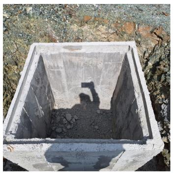
Construction of graded roads has begun but is at initial stages. Drainage chambers will be installed at each lot.
